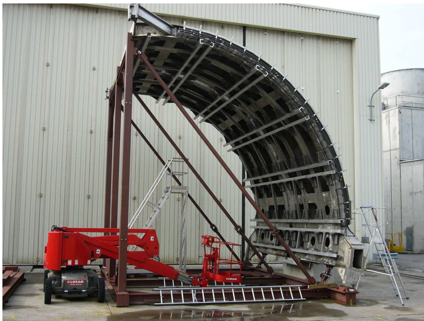
Figure 3.62: EMCAL support structure and the associated rail supports for super modules is shown on its assembly fixture, above ground at the ALICE site (Point 2).
