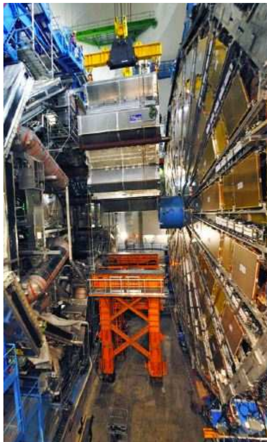
Figure 9.16: Lowering of the first end-cap toroid magnet onto the truck on side A in June 2007. One of the TGC big wheels can be seen on the right of the picture.
